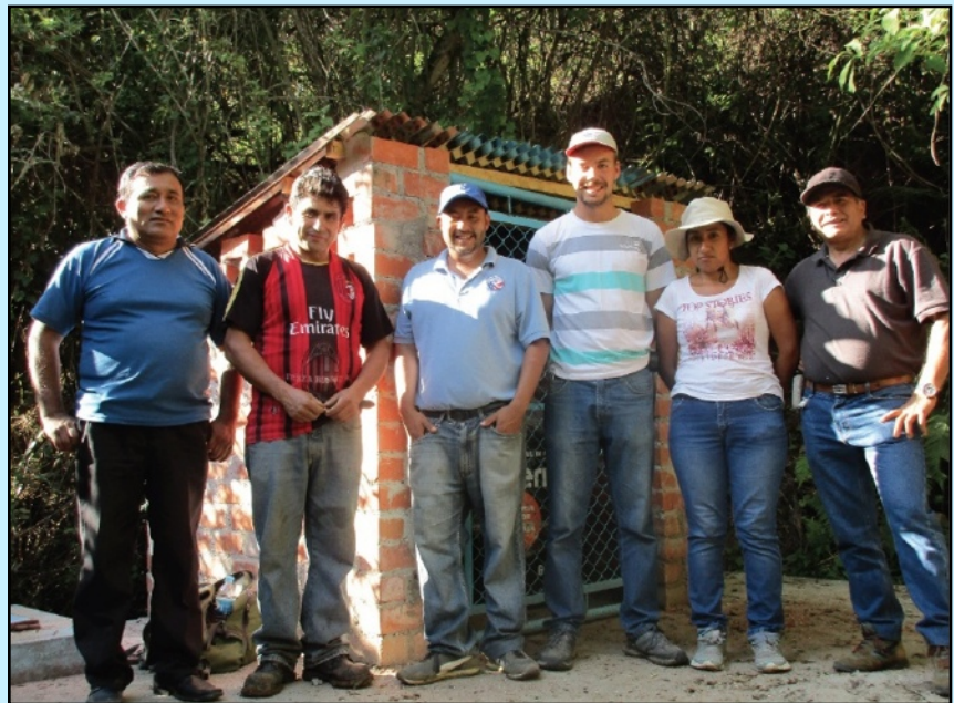
► Posing in front of the chlorination system – which sits on top of the reservoir - are, from left: Head of Environmental Health Department in the Cascas Hospital, community member, PCV Jef Navarette, PCV Leif Hansen, nurse from San Marcos health post, Leif's counterpart in the Municipality.
